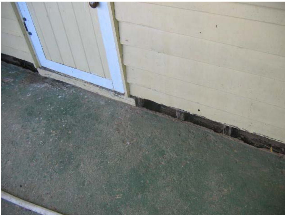
Poor quality concrete at eastern front verandah entrance
