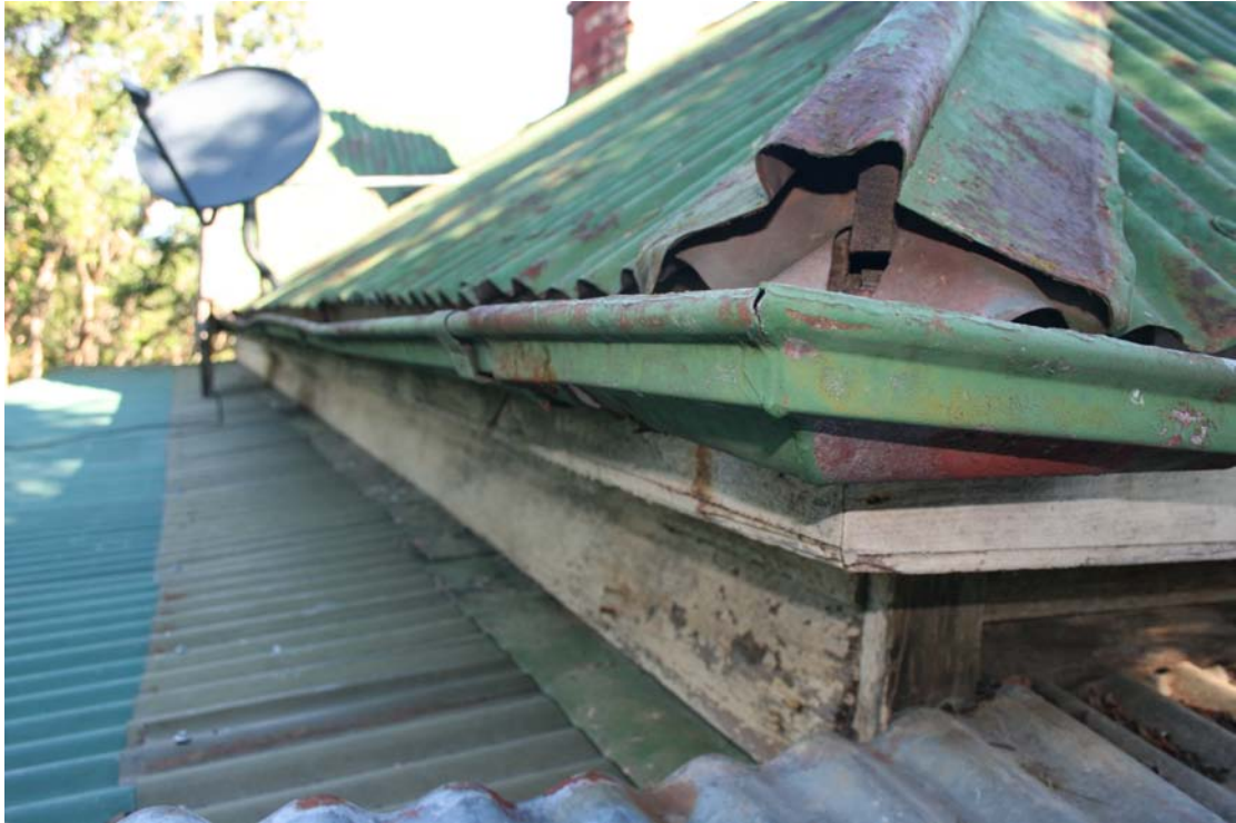
Images show deteriorated gutter, timber elements and corrugated valley tray.
